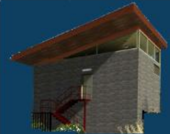
Hope Park Pump CDBG/COB - $800,000
