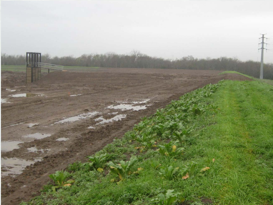
Finished levee – inside PA
