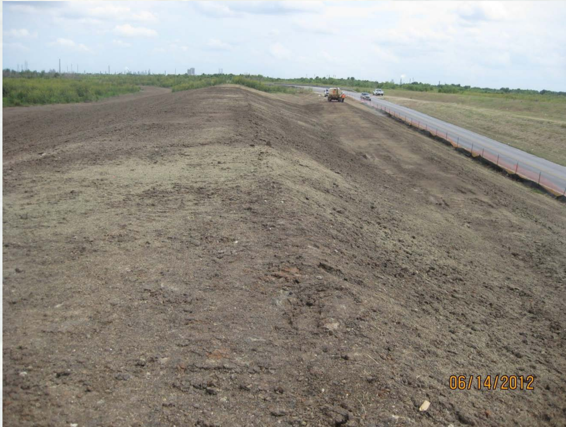
East Cell levee along Mercury Drive
