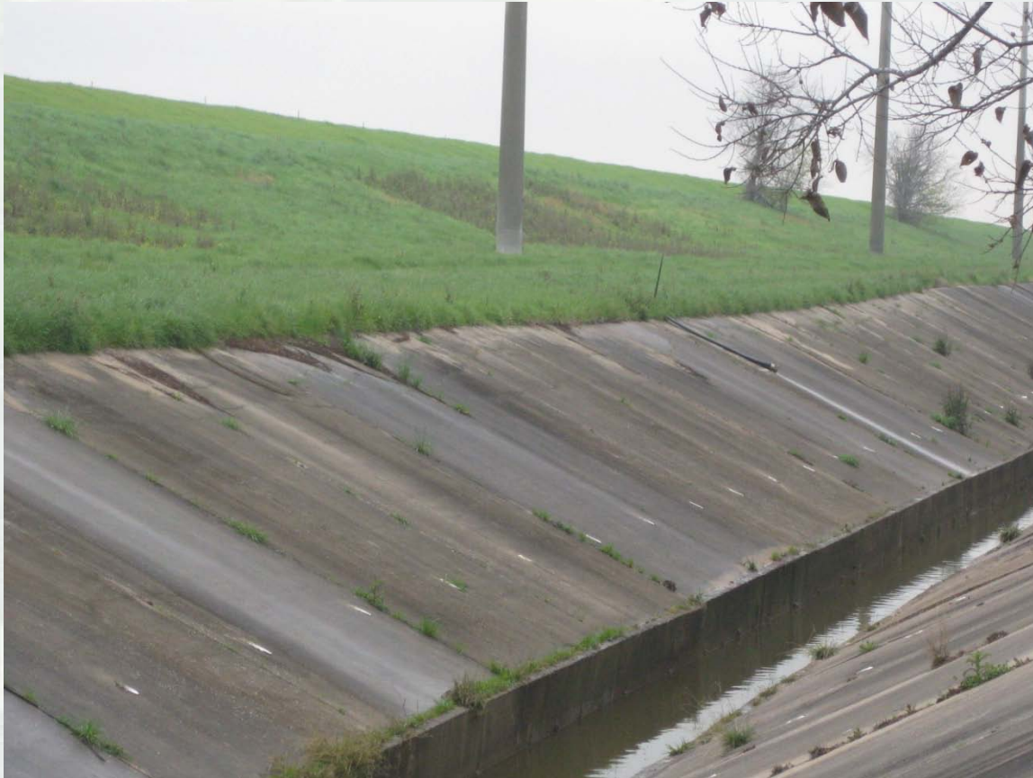
Finished levee – outside PA
