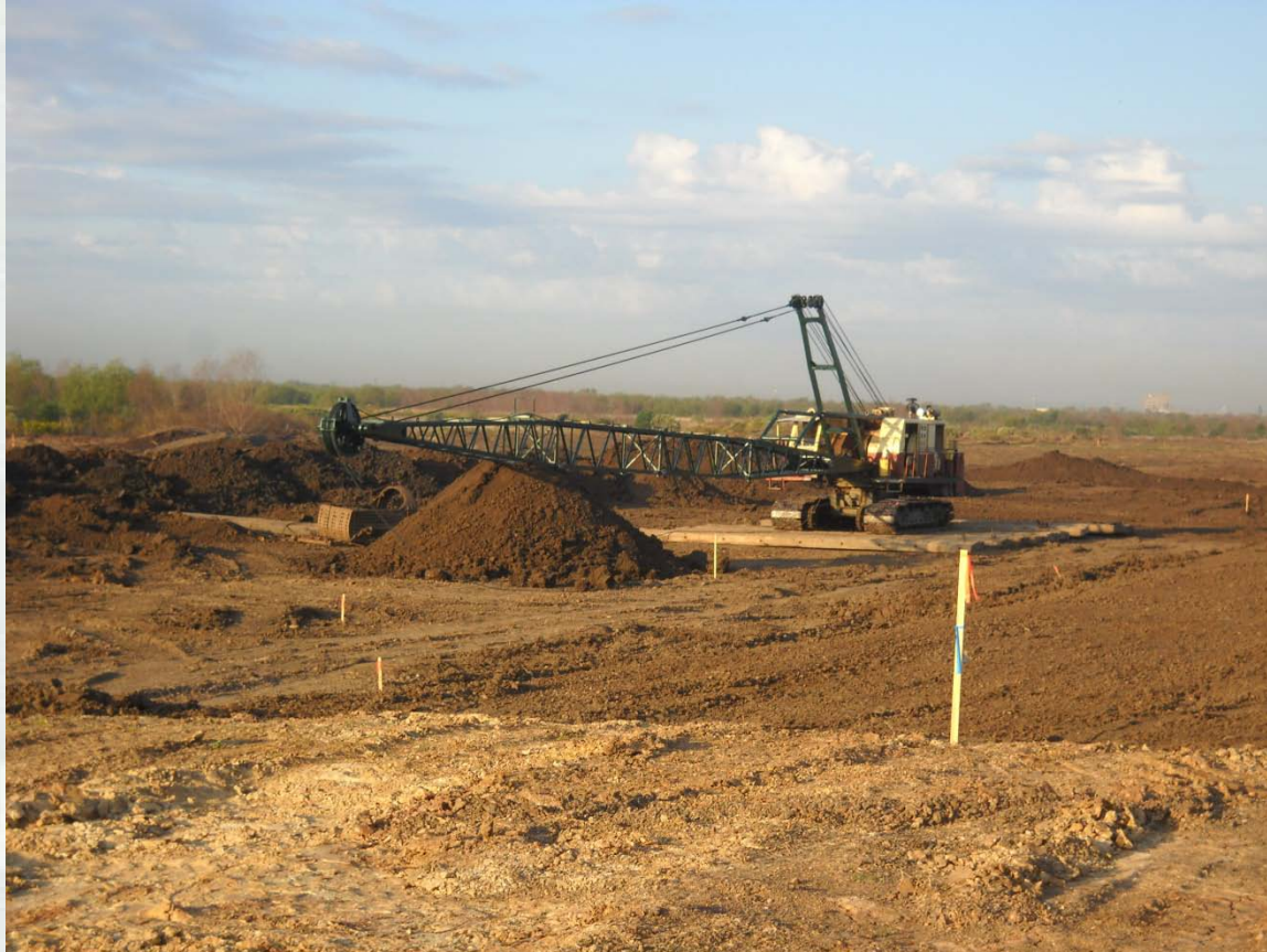
Borrow pit for levee fill
