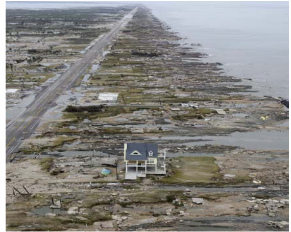
Aftermath of Hurricane Ike to the Texas Gulf Coast near Pelican Island
