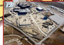
Fort Hood Hospital
