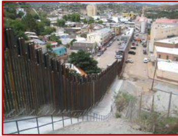
Nogales, Ariz., Border Fence Replacement
