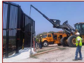
Eagle Pass, Texas, Border Fence Construction
