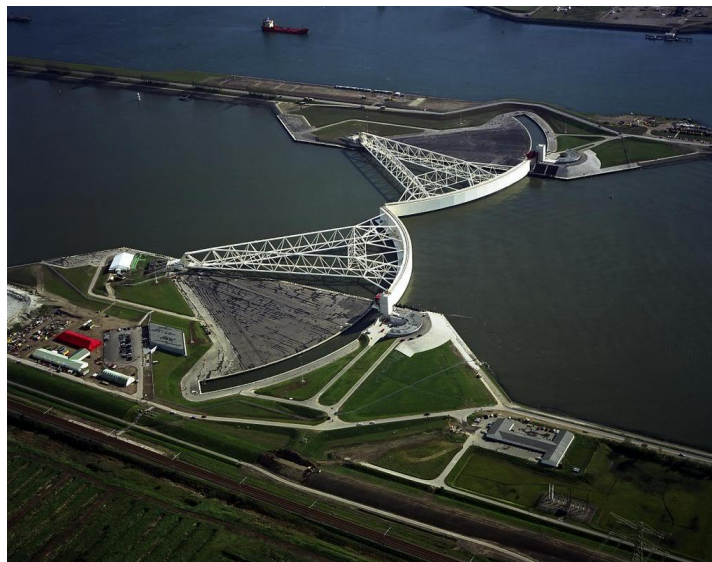
Figure 5-1. Maeslantkering Closure Structure, Netherlands
