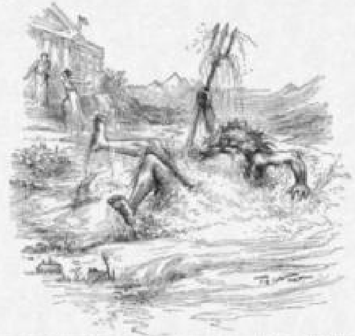
THE NAVY MAKING THE FEDERAL GOVERNMENT'S PROTECTION FROM THE TROUBLE. ESTABLISHED UNDER MANAGER.
