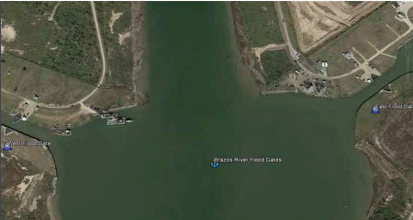
Figure 6. Aerial View of the Brazos River Floodgates.
