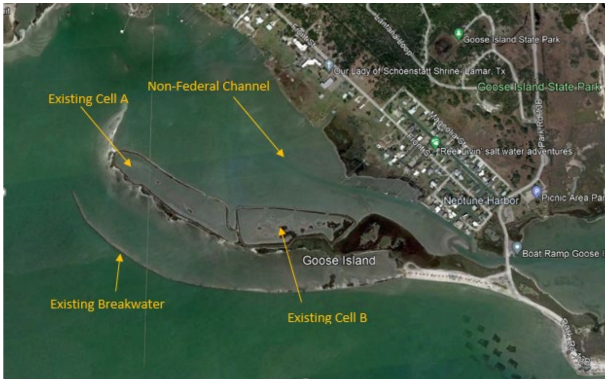
Figure 10. Existing conditions at the proposed site.
