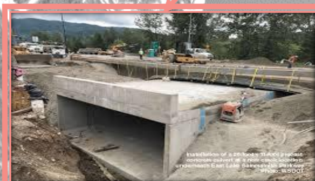
Shallow Section (16 Pre-cast monoliths)
