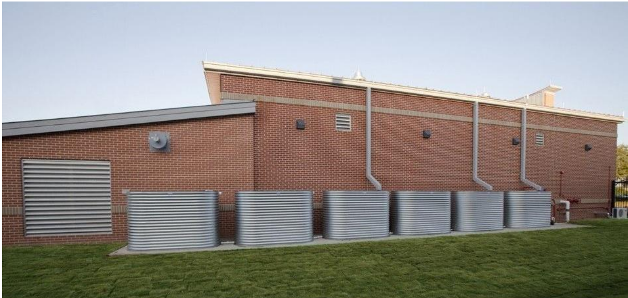
Figure 15. Rainwater harvesting with cisterns at Houston Fire Station #90 (Source: HGAC Designing for Impact).
