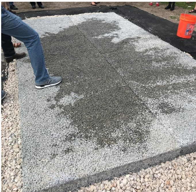
Figure 16. Pervious concrete example during installation. (Source: Molly Ross, 2018)
