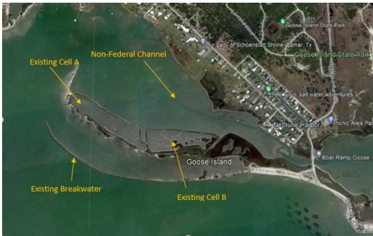
Figure 10. Existing conditions at the proposed site.
