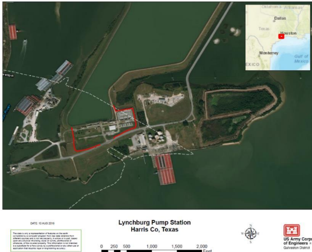
Figure 1-4: Lynchburg Pump Station
