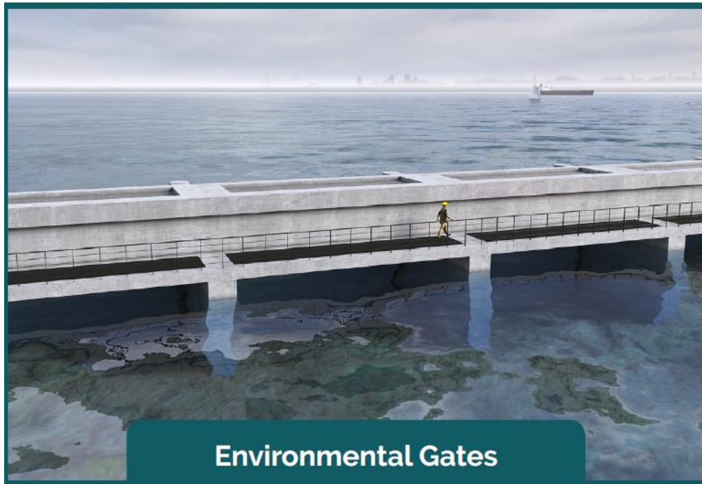
Figure 6-9: Shallow Water Environmental Gates (SWEG) (Conceptual Rendition)
