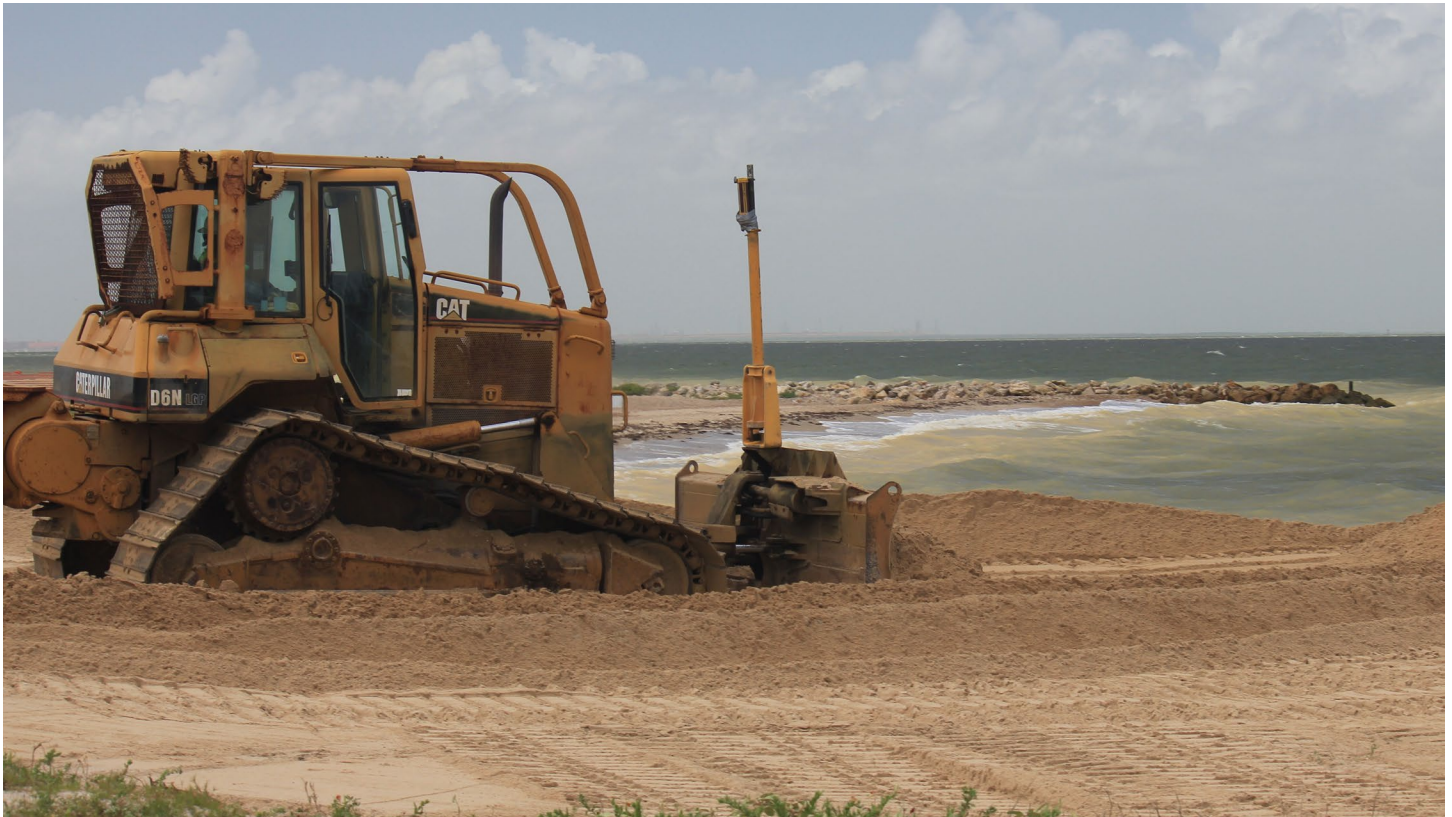
Example of beach renourishment in-progress
