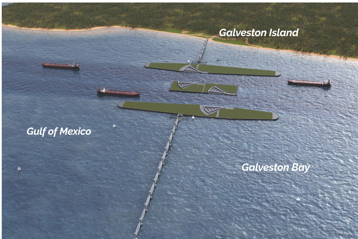
Conceptual rendering of the proposed sector gates at the Bolivar Roads Gate System
