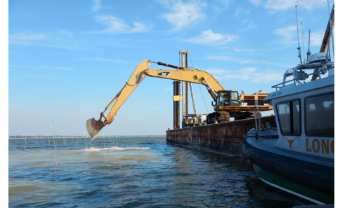
Photo of a barge placing material for oyster reef creation
