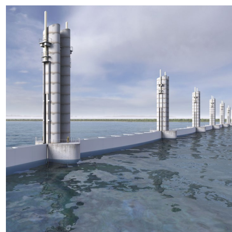
Figure 3.21: Location and conceptual rendering of the vertical lift gates in the open (top image) and closed (bottom image) positions.
