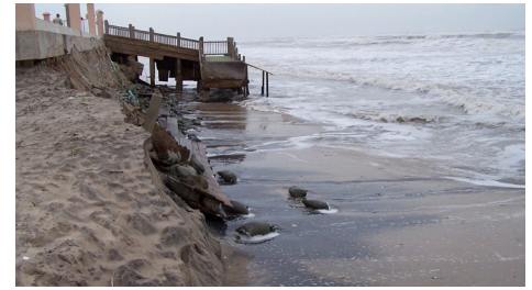
Photo of shoreline erosion on the Texas coast
