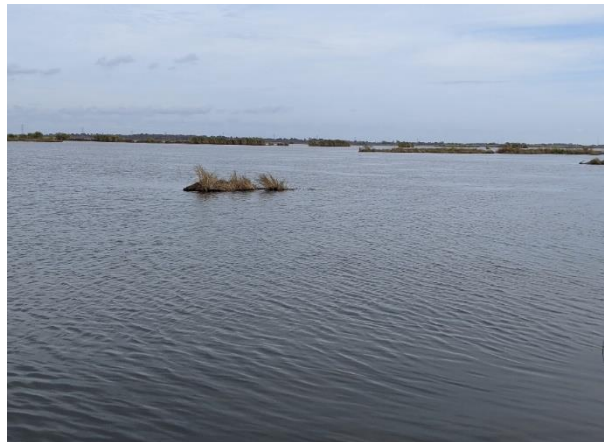
Figure 8. Open water landward of the containment dike
