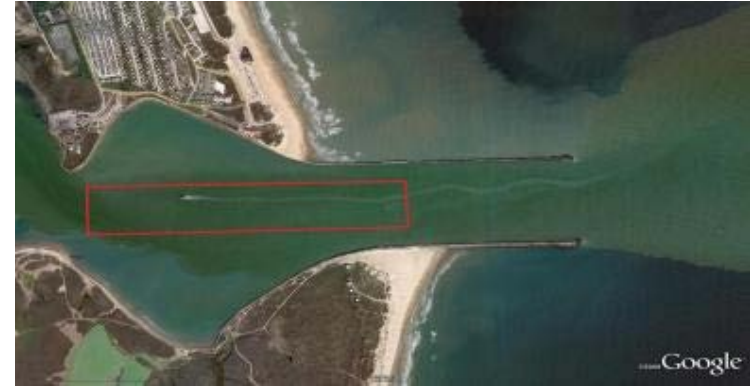
In-channel Sediment Trap (holds 200,000 cy of material)
