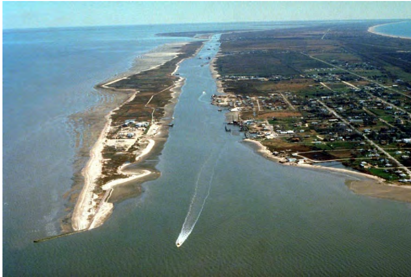
Figure 1-2 – GIWW Opening at Port Bolivar, Texas in 1999
