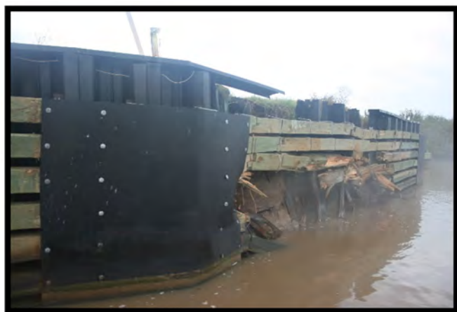
Figure 3-2 – Guidewall Damage from Barge
