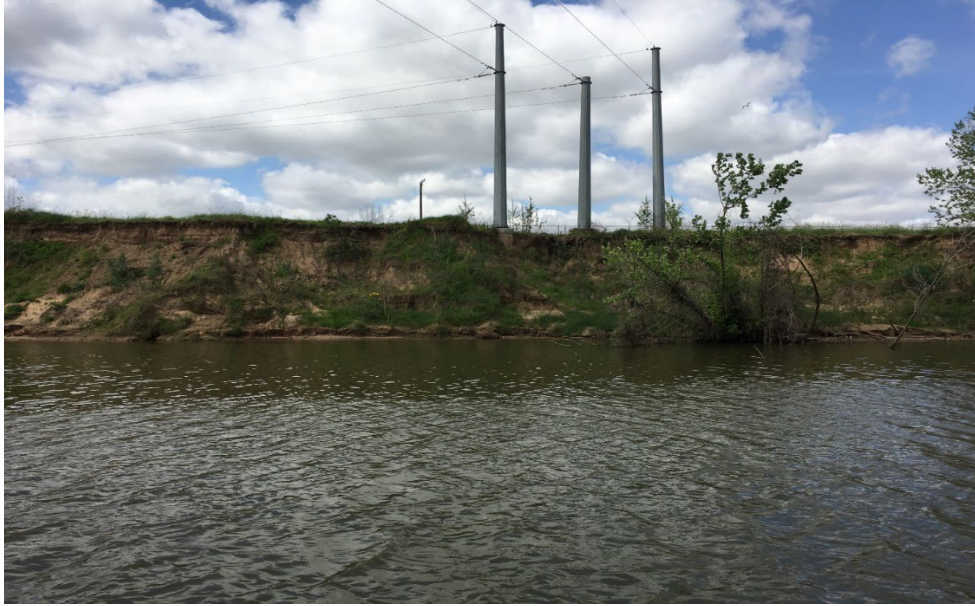
Figure 1-4: Exposed Power Transmission Poles near Mary Rhodes Pump Station
