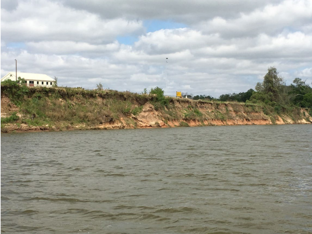
Figure 1-6: Erosion along the Colorado riverbank at Mary Rhodes Pump Station
