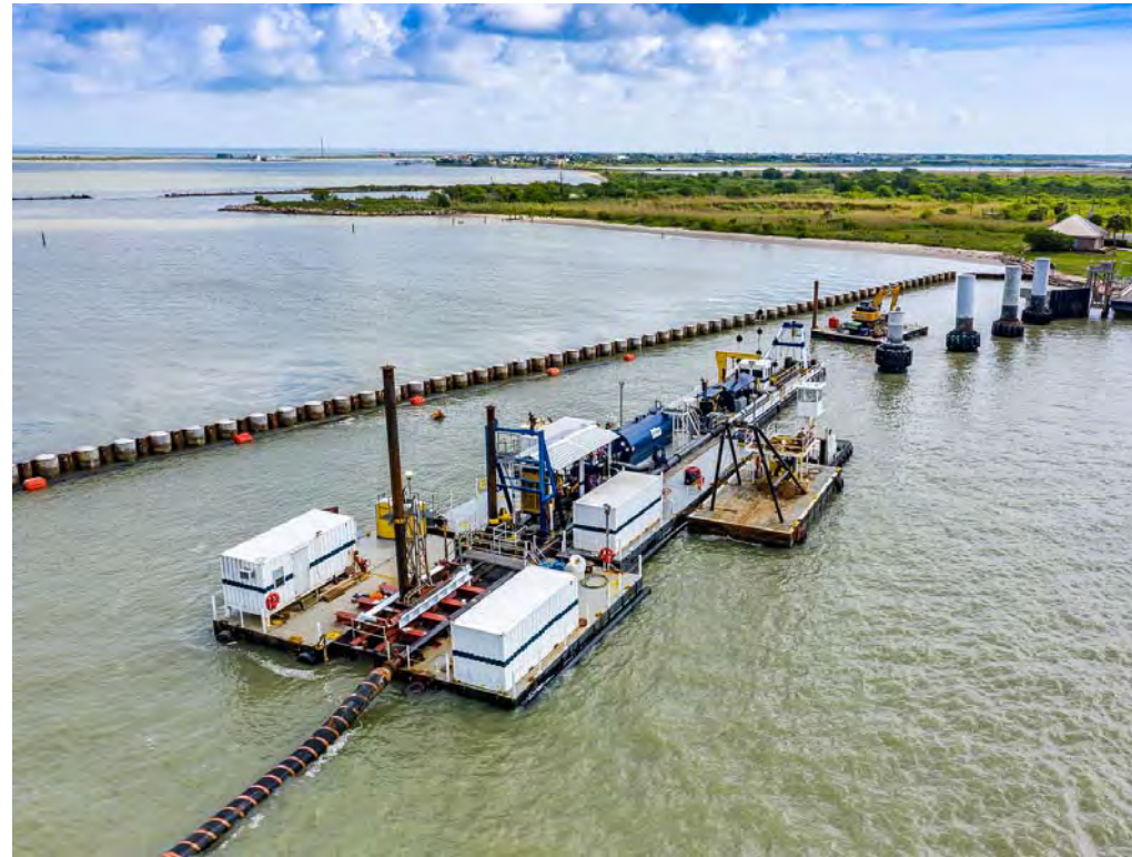
18" General Pershing at the Texas Department of Transportation Bolivar Ferry Landing Maintenance Dredging
