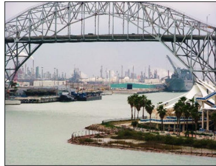
Petrochemical Facilities at Port of Corpus Christi
