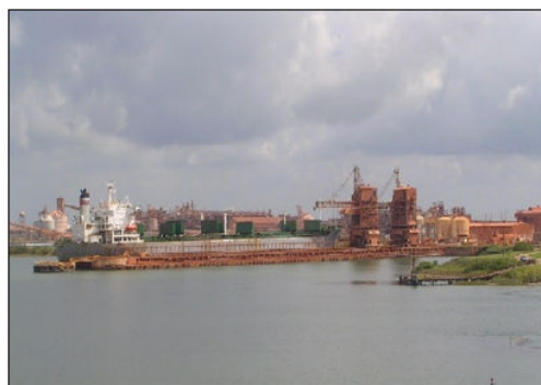
Alcoa Bauxite Discharging Berth at Point Comfort
