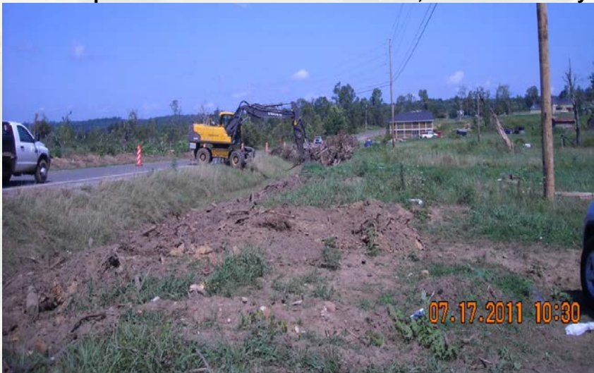
17 July 2011 – Ineligible Debris Being Removed by the the Corp's Contractor off ROW HWY 117, Jackson County
