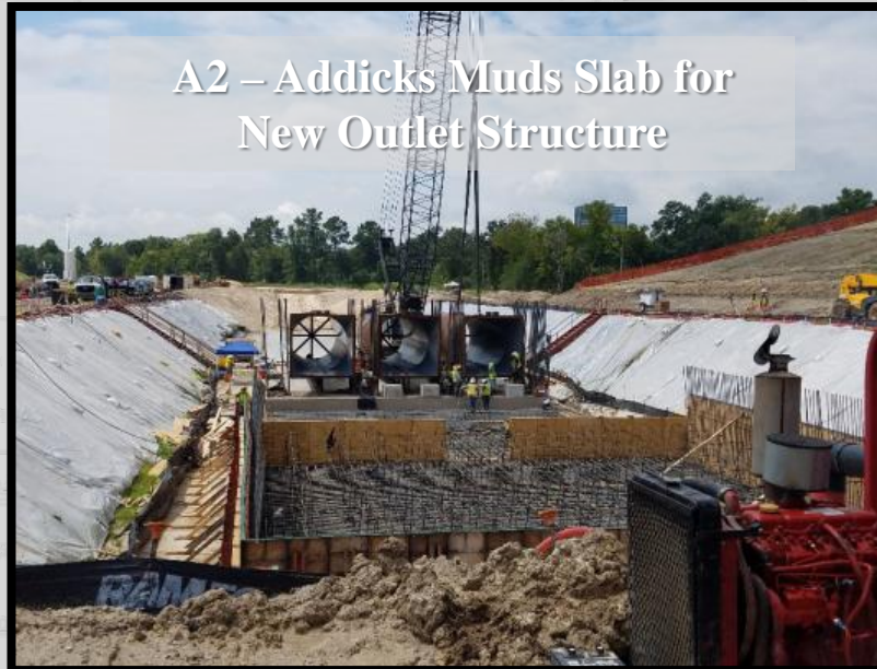
A2/A3 - Addicks Cofferdam, Primary Excavation and New Outlet Channel Area
