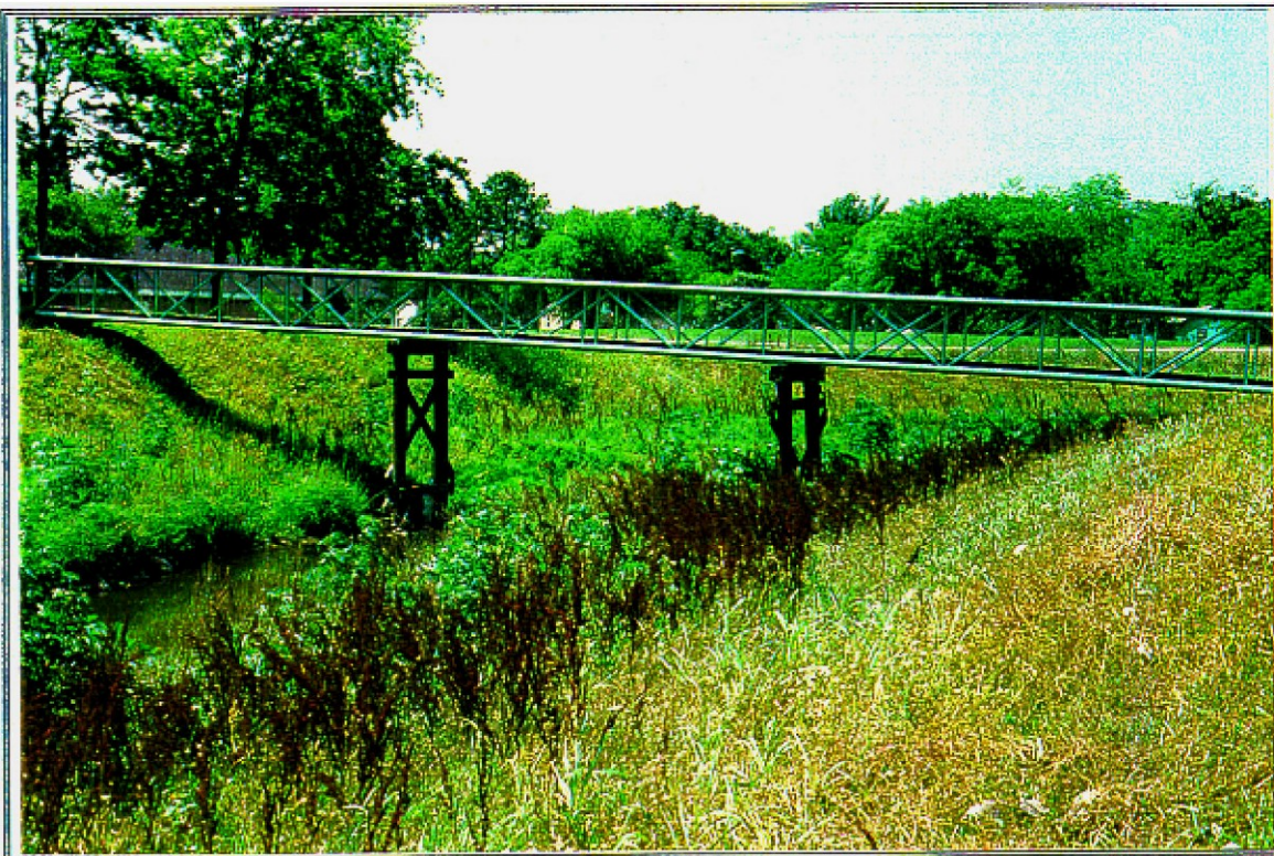
N = 0.05: Looking downstream at pedestrian bridge in Hutcheson Park.
