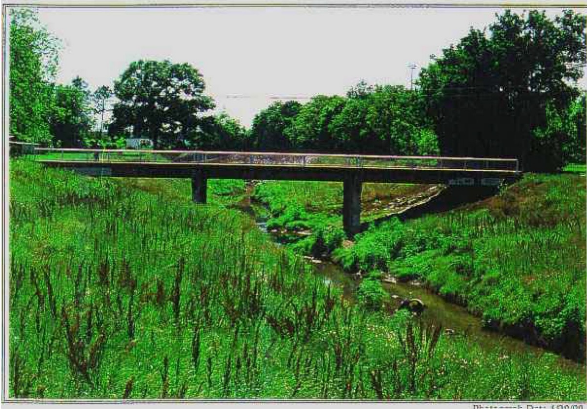
N = 0.05: Looking upstream at bridge on Manitou Street.
