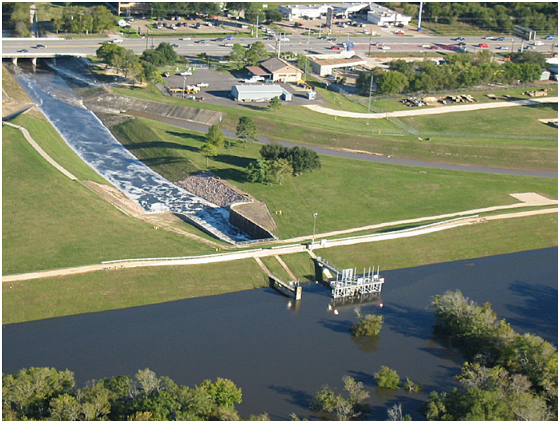
Figure 5 – Aerial View of the Outlet Works
