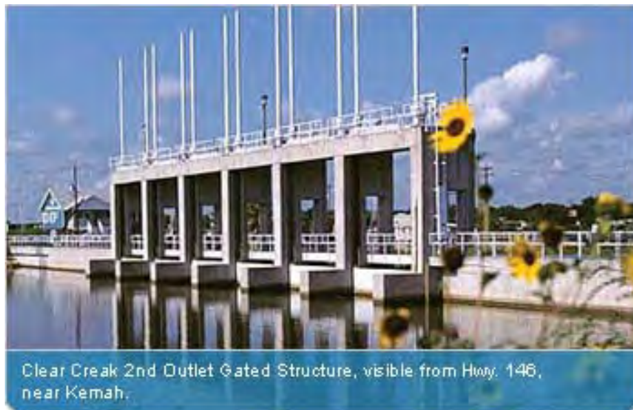
Figure 7 – Photo of Second Outlet and Gate Structure
