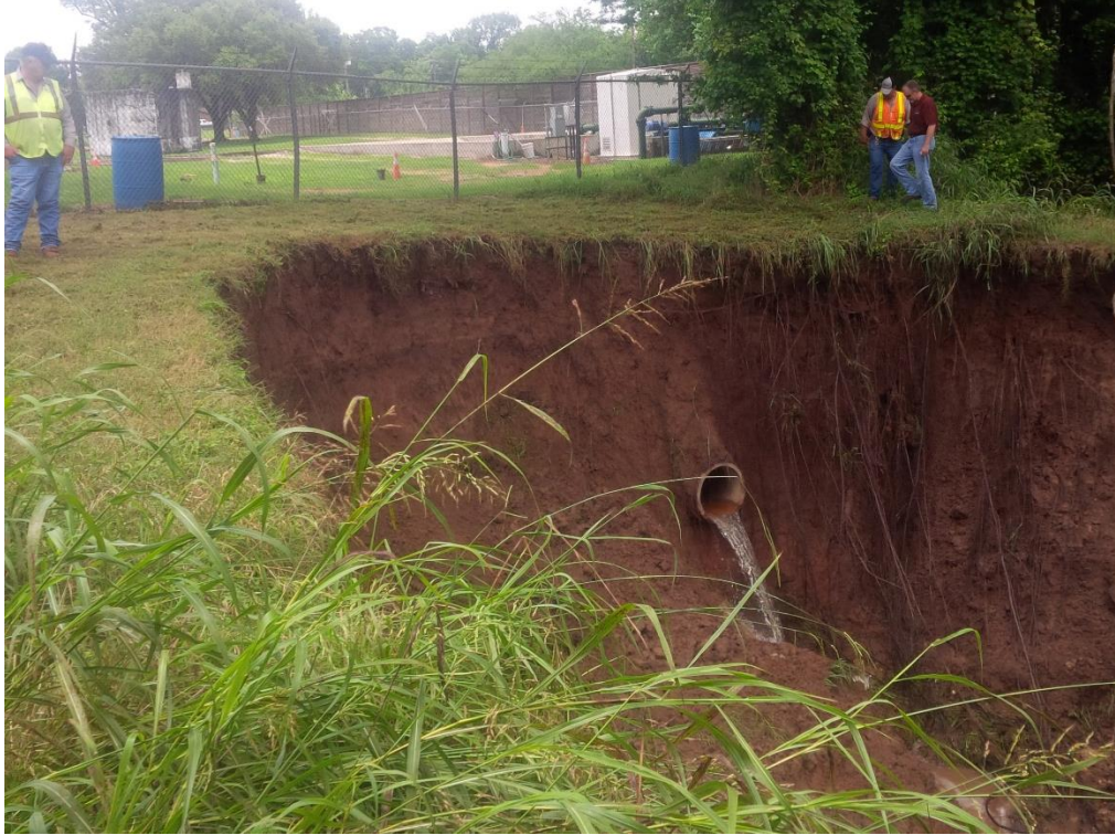
Figure 2: Site conditions during a May 2016 site visit
