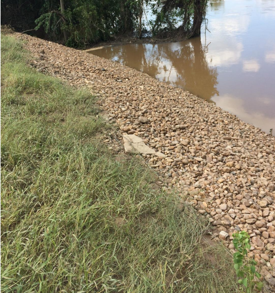
Figure 4: Temporary repair completed in 2017 prior to Hurricane Harvey
