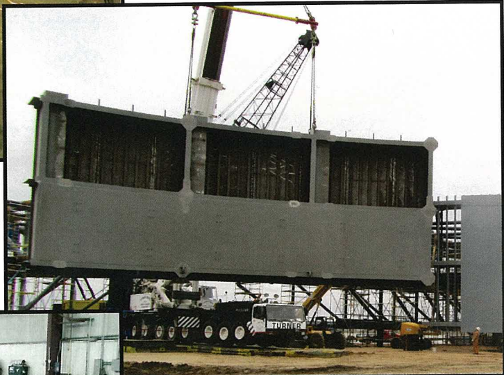
66 Ton Gate Truss In Fabrication
