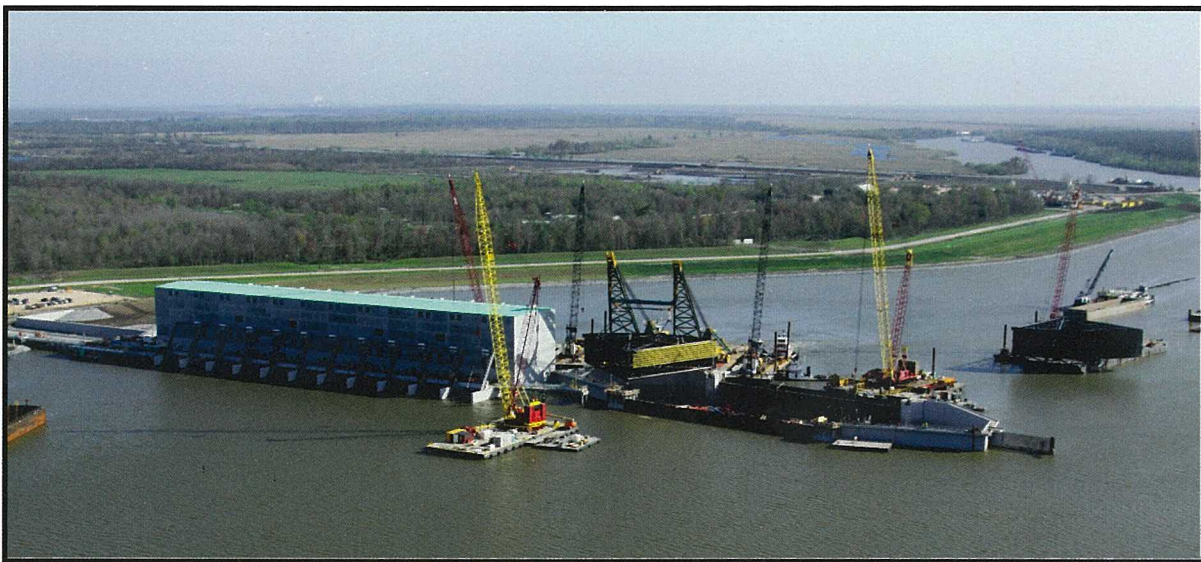
West Closure Complex Project, Southwest of Belle Chasse, Louisiana
