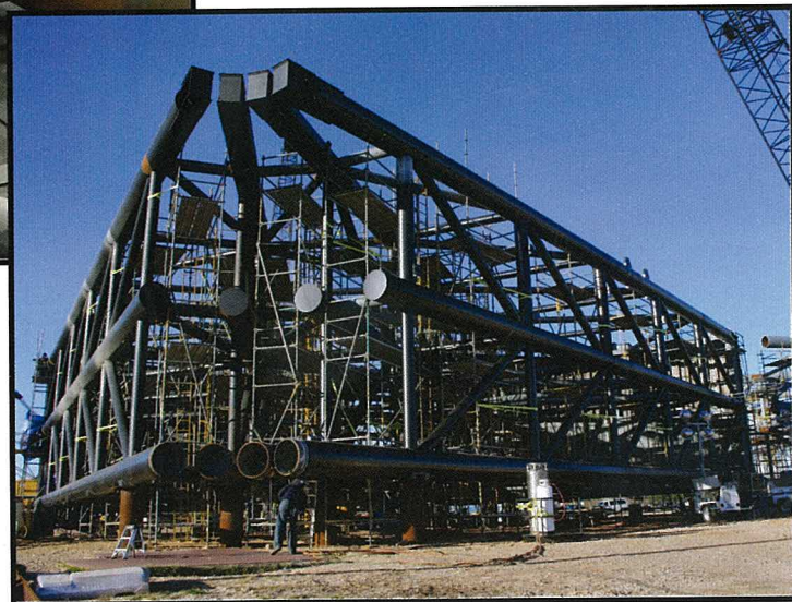
66 Ton Gate Truss In Fabrication
