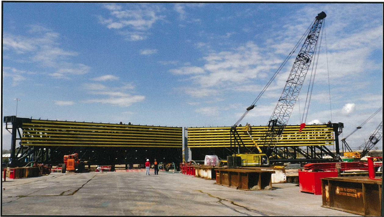
Completed Gates Ready to Load on Barge
