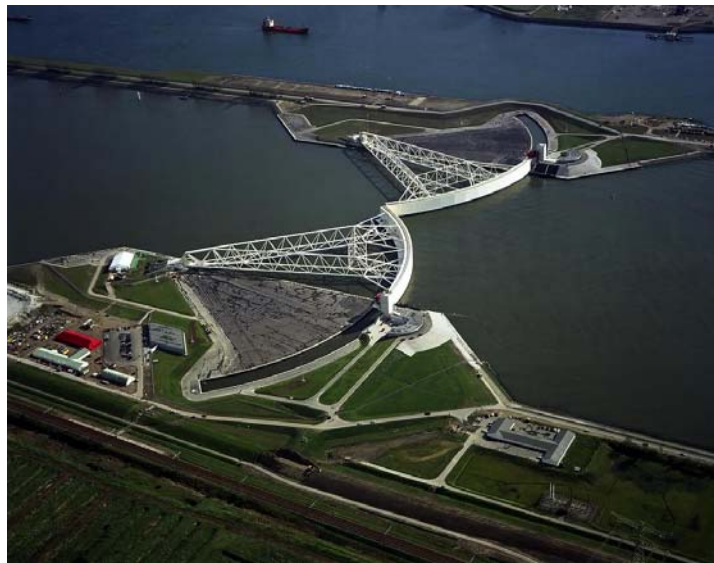
Figure 5-1. Maeslantkering Closure Structure, Netherlands
