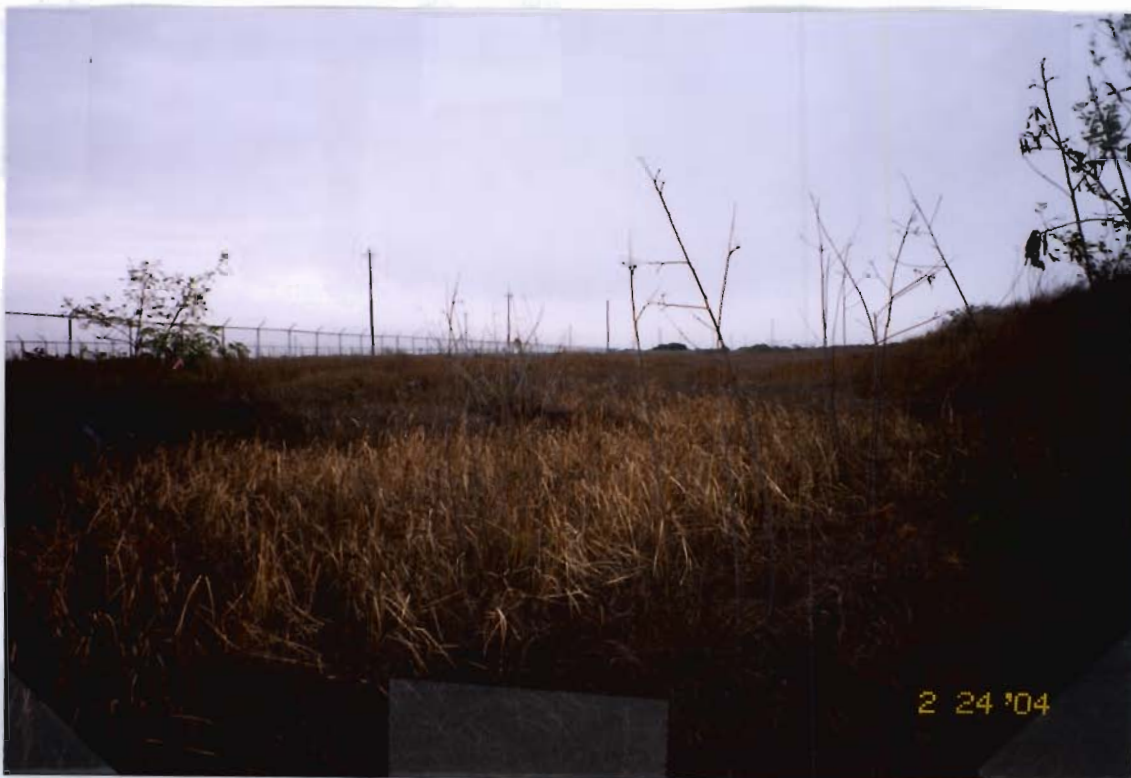
Photo 4: Facing NE along borrow area for levee along north property line to show cattail wetland resulting from water trapped by depressional area between levee on the right (south) and roadbed to the left (north).
