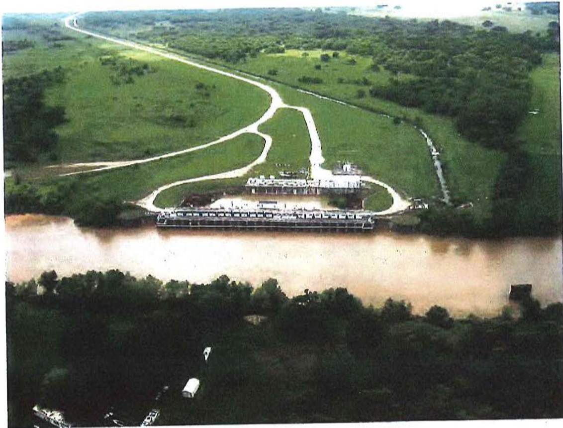
Figure 3: South Texas Project Reservoir Makeup Pumping Facility Aerial Photo Looking West
