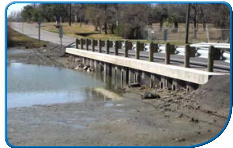
After "coffer dam" removed
