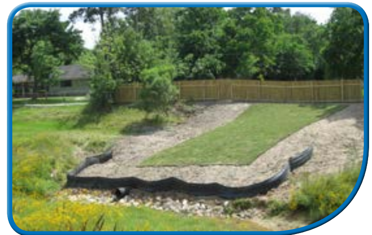
Side slope and outfall after maintenance
