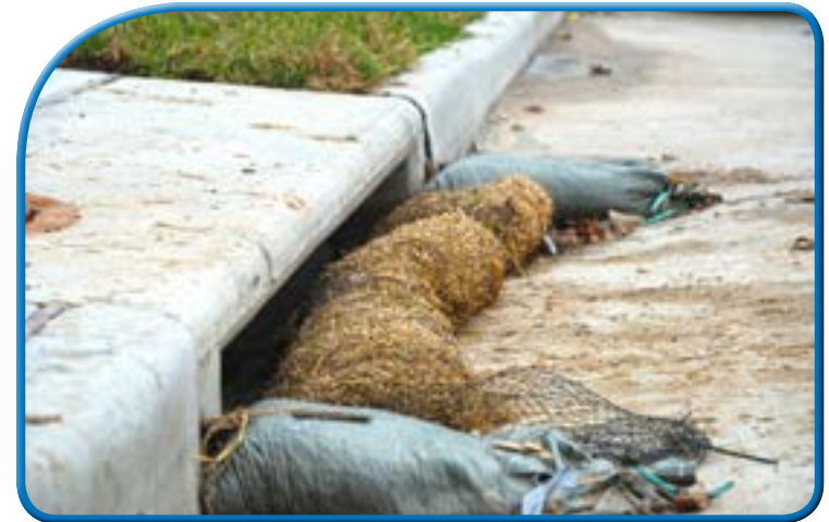
Intake protection barrier
