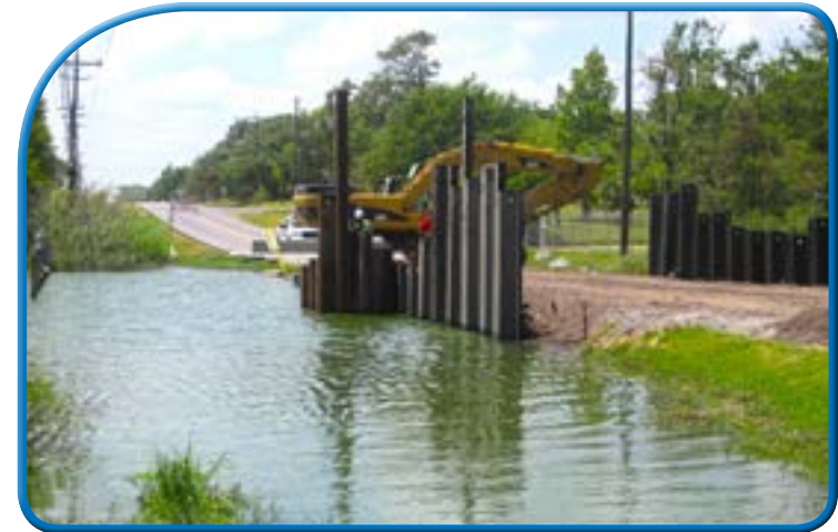
Use of "coffer dams" during construction
