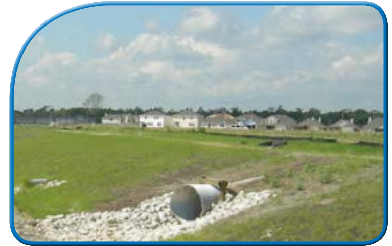
Example of outfall after maintenance
