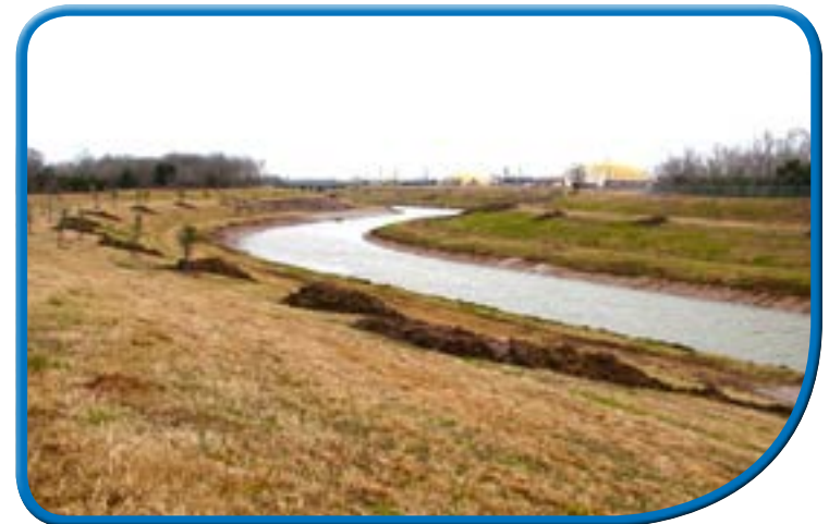
Existing Drainage Ditch
