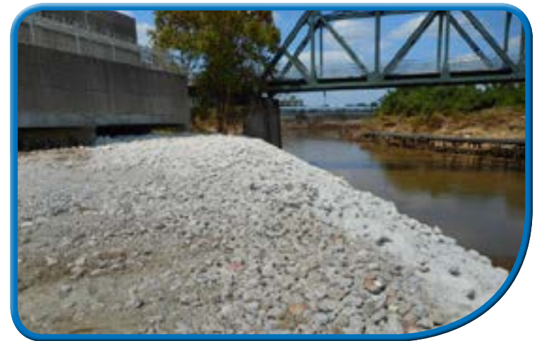
After damage repair
