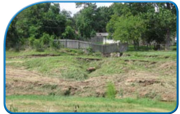
Side slope and outfall before maintenance
