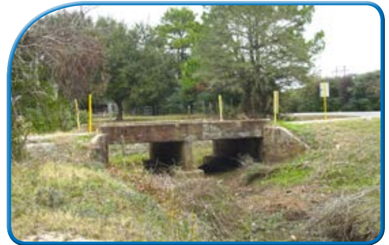
Bridge before improvement
