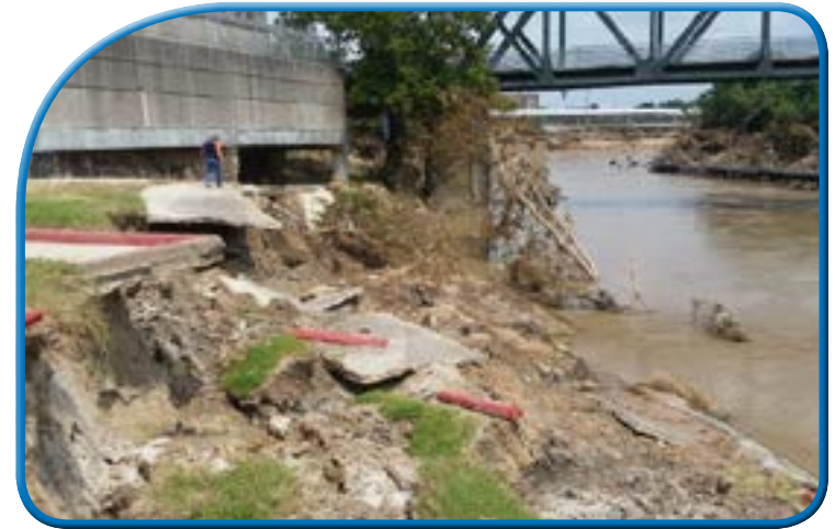
Before damage repair
