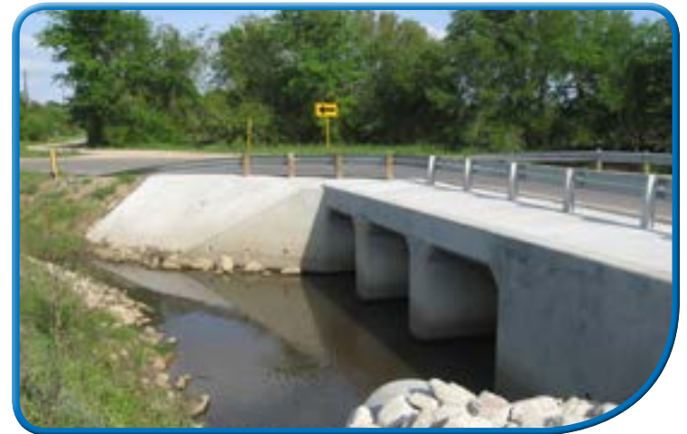
Bridge after improvement
