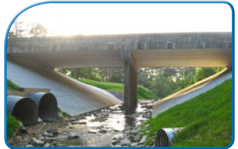
Outfall structures adjacent to channel
