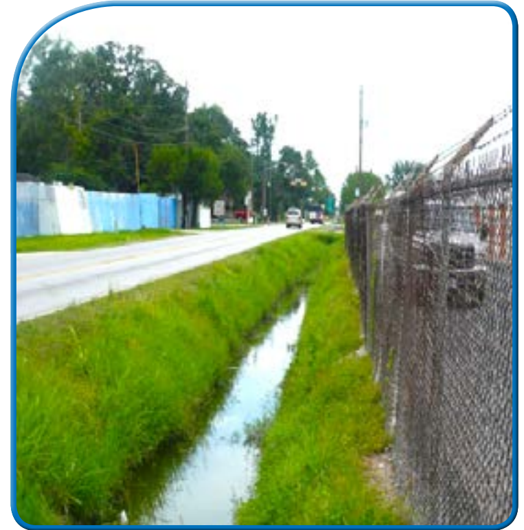
Ditch constructed in uplands
