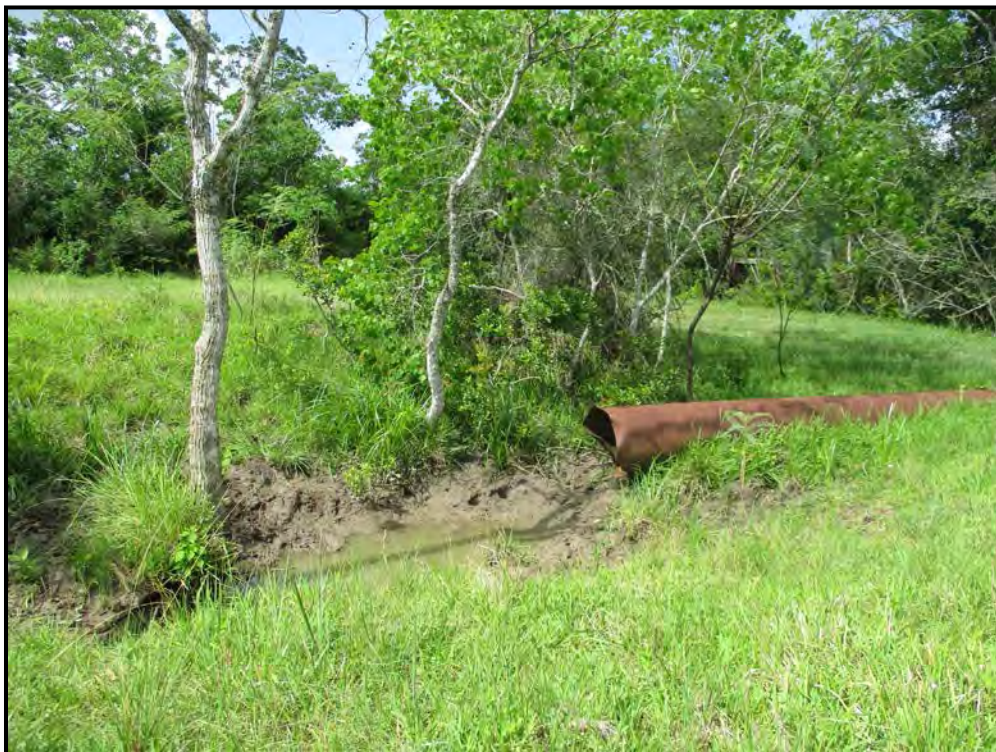
Photograph 8 – Culvert at western edge of man-made drainage ditch
