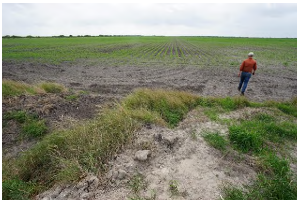
Photo of Blow Out in Existing West Main Ditch After Large Rainfall Event
