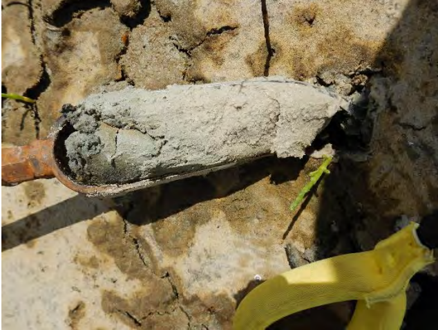
Picture 13: RW02BPH Bearing: N/A Date: 5/7/2021
