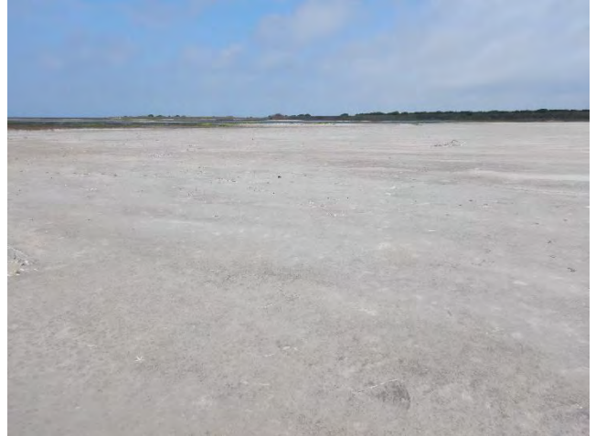
Picture 20: RW03BPH Bearing: West Date: 5/10/2021
