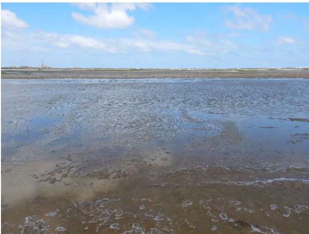
Picture 11: RW02BPH Bearing: East Date: 5/7/2021
