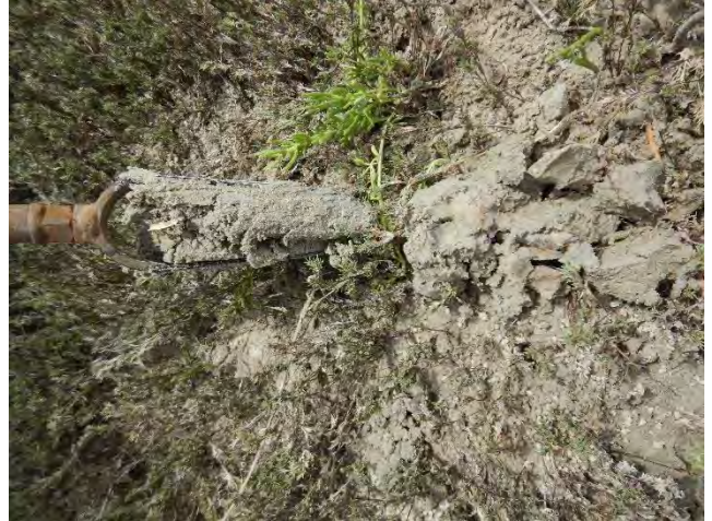
Picture 8: RW01BPH Bearing: N/A Date: 5/7/2021
